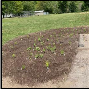
The Finished Rain Garden
